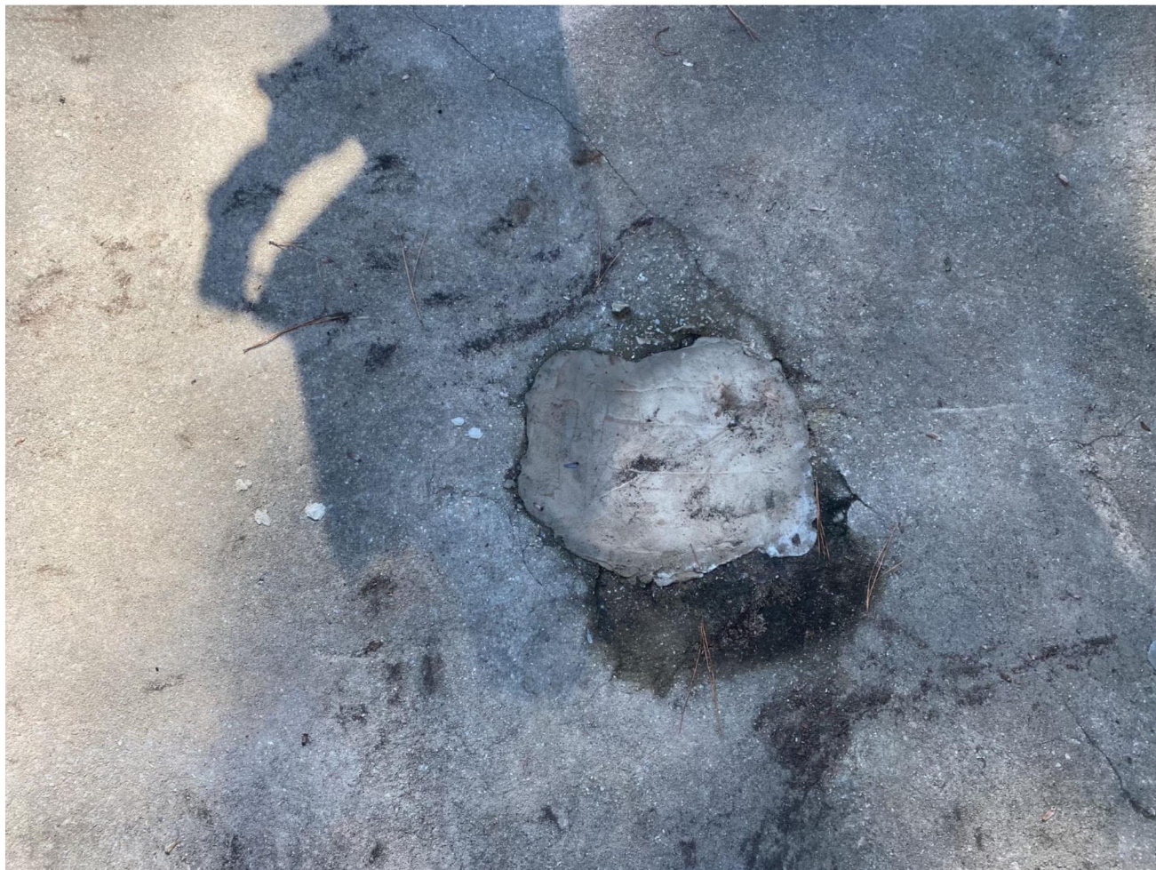
Photo 3 of 3, December 5, 2023, RCRA Cap surface spalling spot cleaned out and repaired, located near the north edge.
