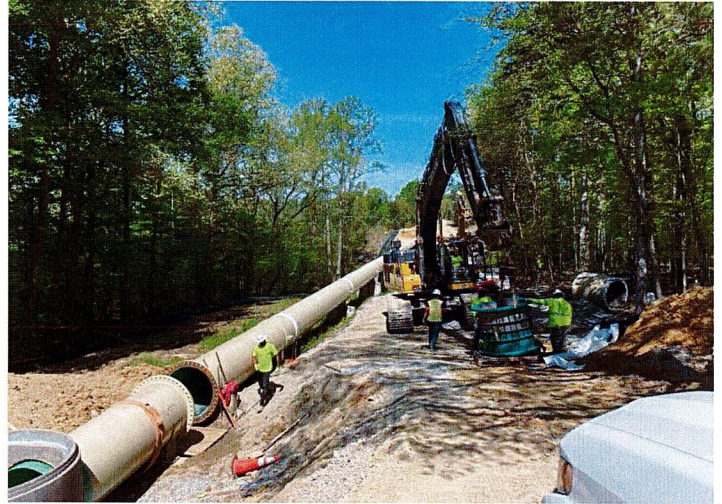
(Above) – Construction of the Richland Creek Sewer Aerials
