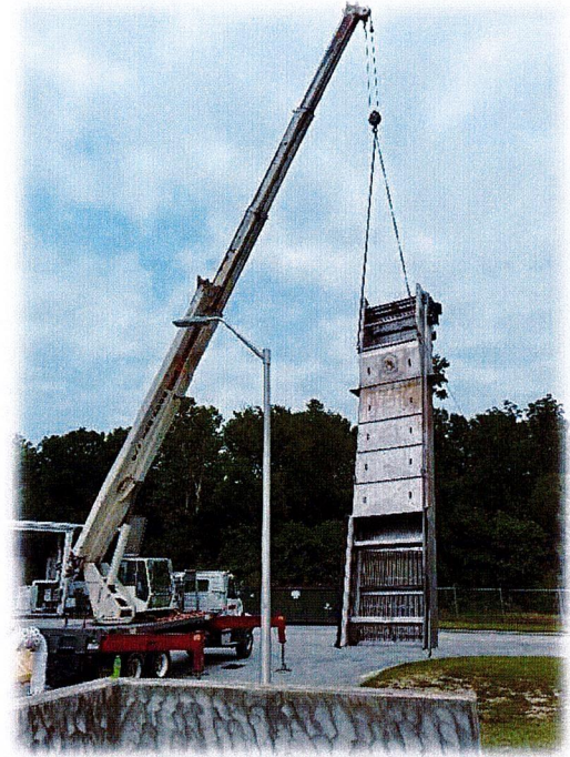
(Right) – Coarse Barscreen being removed for repair
