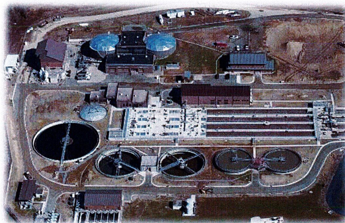
(Above) – Aerial view of Westside WWTP
