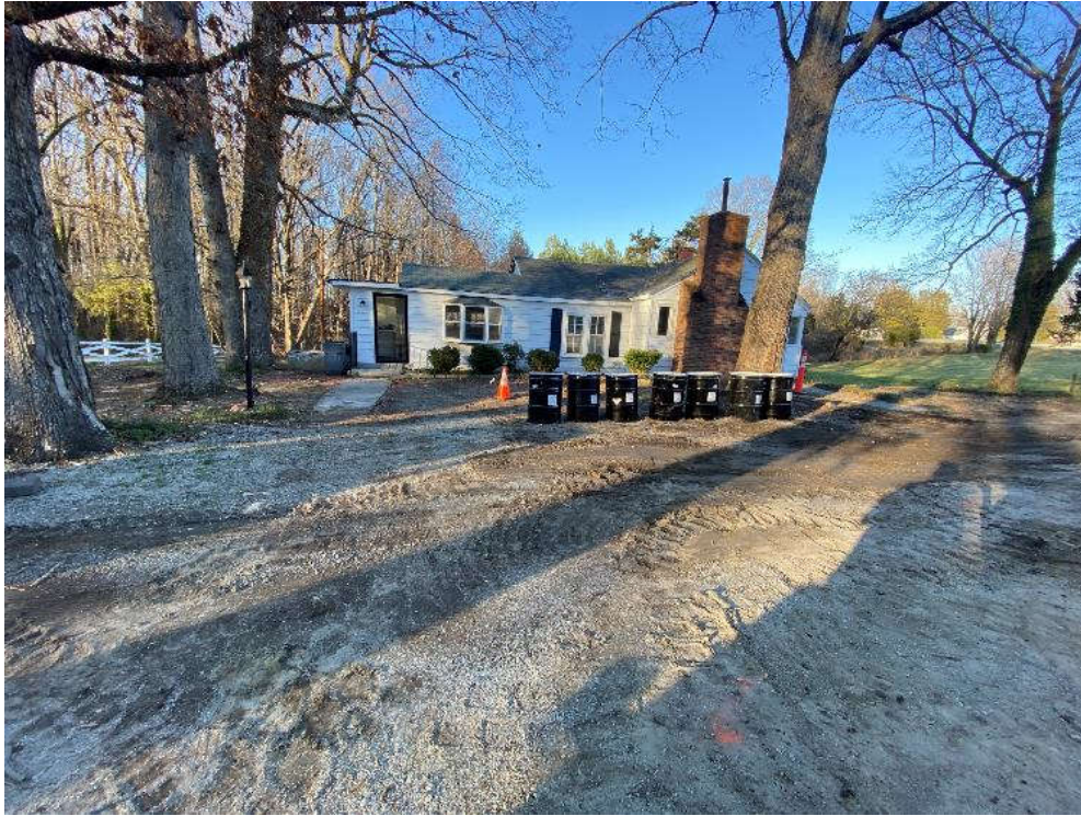
Photo #15: IDW Location
